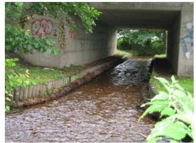
(8) A rough gravel bed and berms on either side improve passage under a bridge
