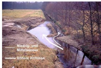
(5) A sand trap holds back eroded material, and alders shade the streambed, prevent mass growth of aquatic and marsh plants and protect the bank
